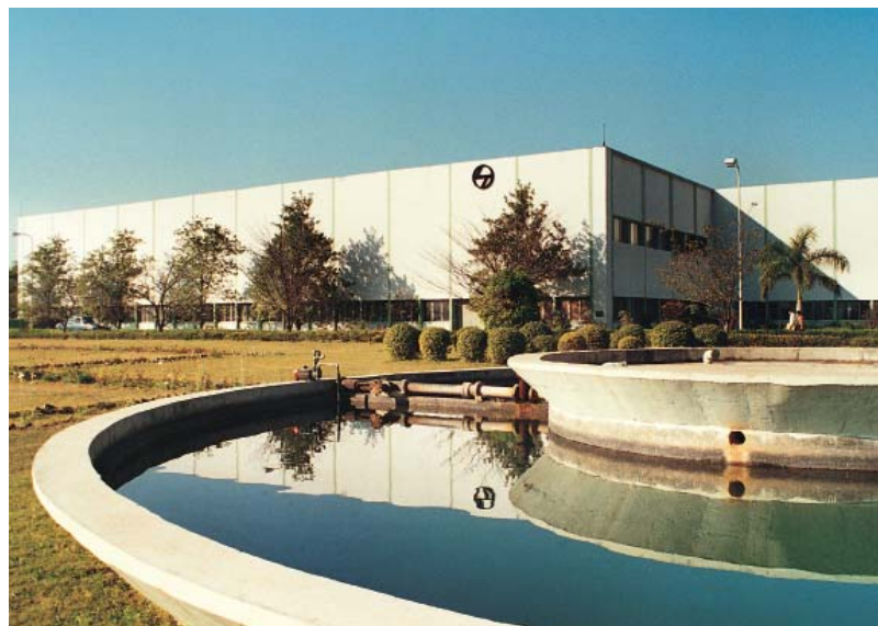
Switchgear Factory, Ahmednagar
