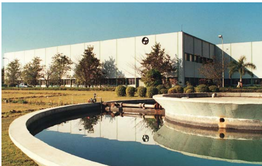
Switchgear Factory, Ahmednagar
