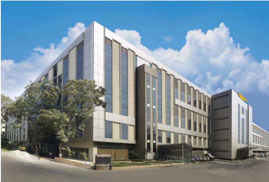
Switchgear Factory, Mumbai
