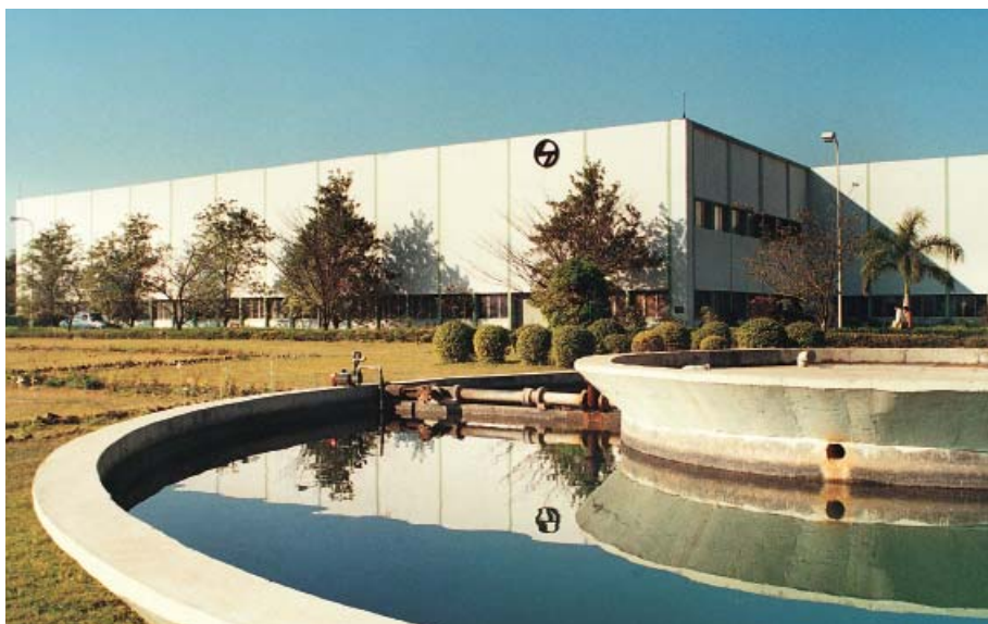
Switchgear Factory, Ahmednagar
